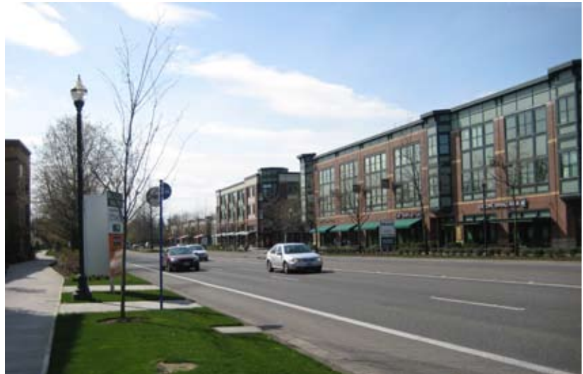
Most of the retail is oriented toward Cornelius Road, a main arterial road that runs through the project.
